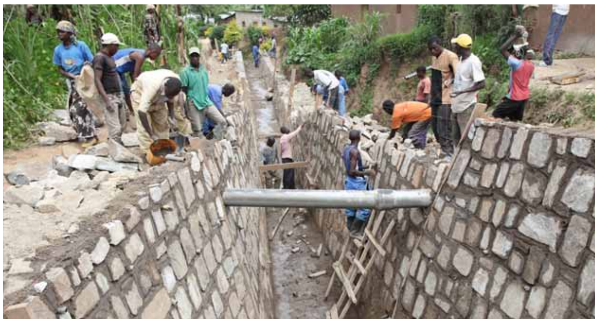
Construction of water drainage that is supported by UN-Habitat and ONE UN in Bugesera, Rwanda. © UN-Habitat /Julius Mwelu
